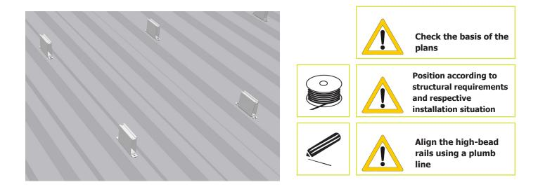
Attach the high-bead rail with the sheet metal screws. Use 2 sheet metal screws per high-bead rail. To prevent water from penetrating between the high-bead rail and the roofing, the high-bead rail must always be mounted on a raised corrugation. The base of the high-bead rail as well as HS clamp XL is covered with EPDM sealing strips.
